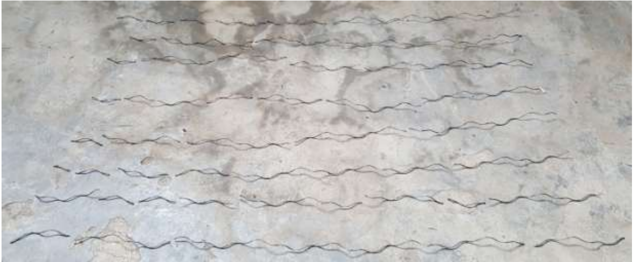
Figure 6. Broken wires of one strand after its unstranding.
