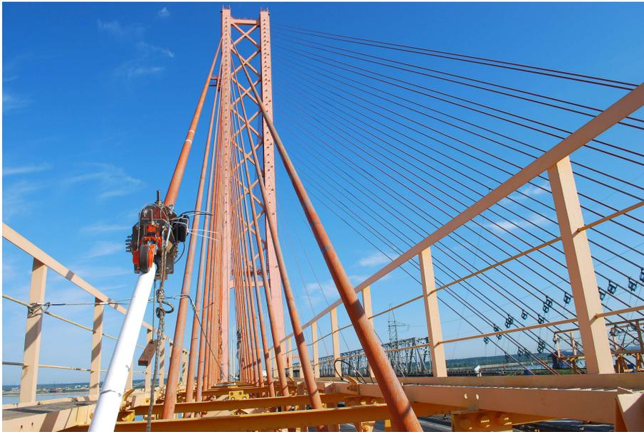
Figure 1: Stay ropes inspection by INTROS device
