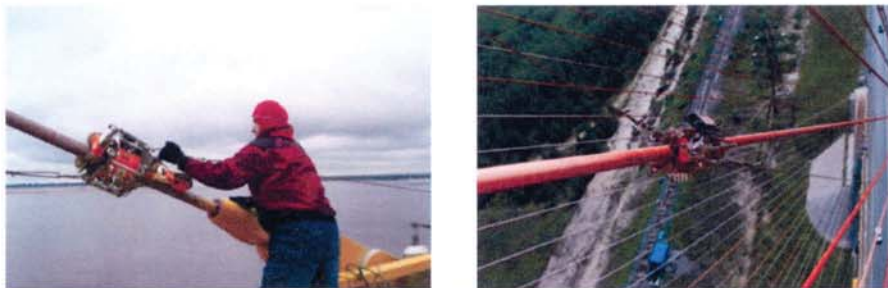
Figure 4: Inspection of a stay cable 72 mm in diameter with MH 60-85.
