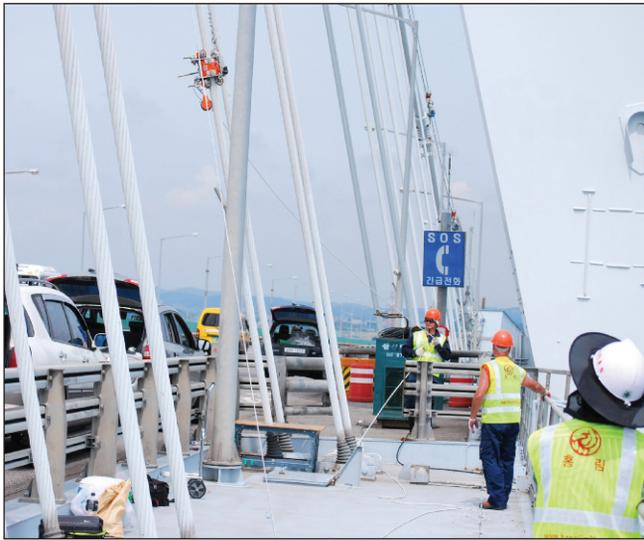
Figure 6. Stay rope testing at the Yeongjong Bridge, South Korea.
