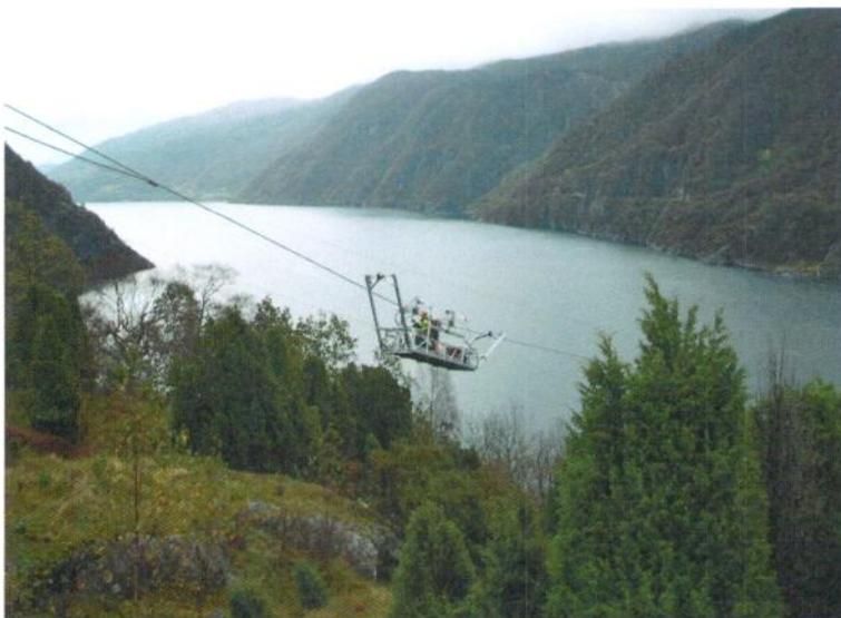
Fig. 19: Inspection of an overhead transmission line conductor over a fiord in Norway.
