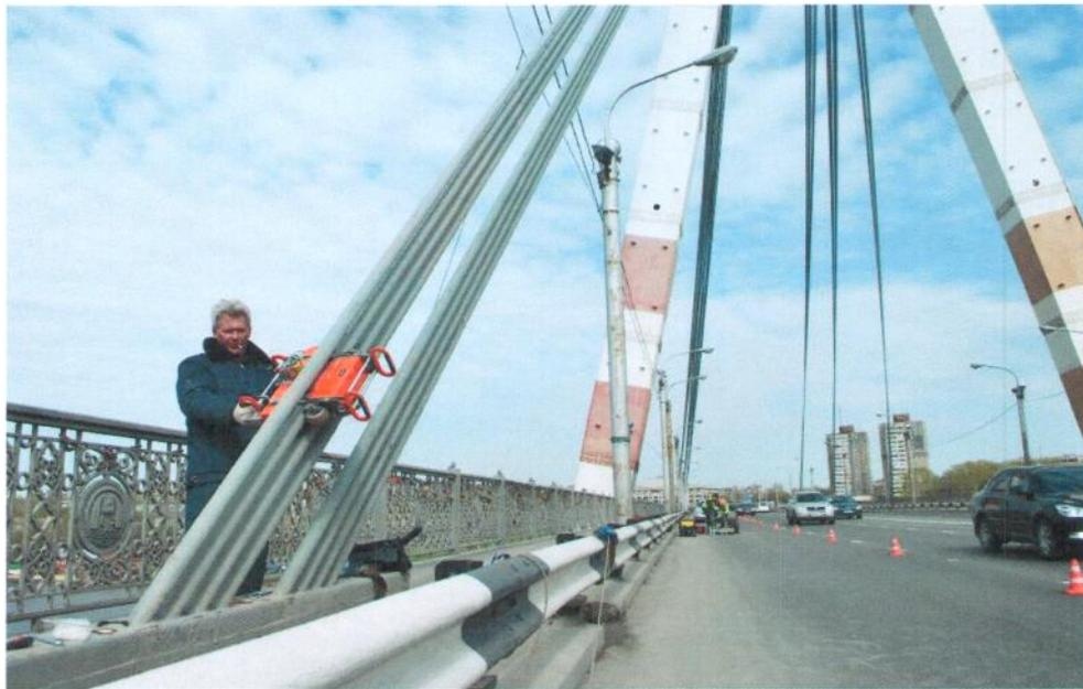
Fig. 18: Magnetic head adopted for close located ropes testing.
