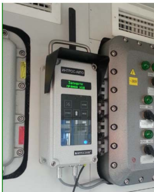
Figure 2: Control and display unit of Intros-Auto in the hoist operator booth
