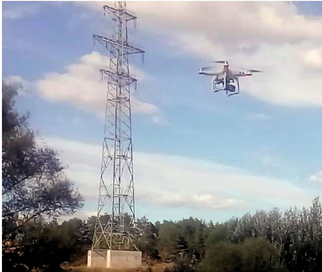
**Fig. 1.** Visual inspection of conductors of 35-kV OHL using a drone with camera.
