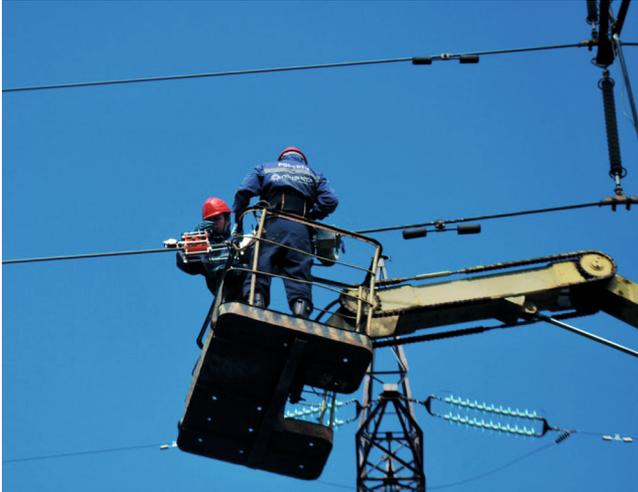
Fig. 3. Installation of magnetic detector on conductor.
