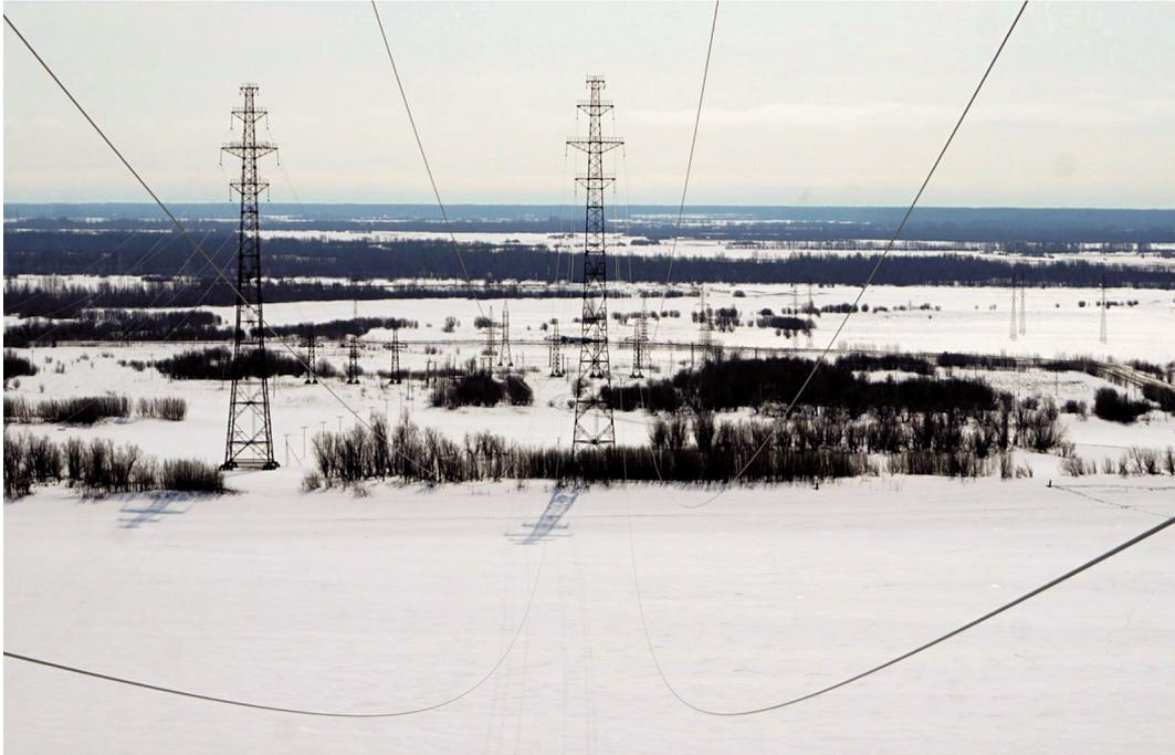
**Fig. 8.** Crossing of the Ob' River by 110 kV Kudelinskaya – Shubinskaya and Roslyakovskaya – Priobskaya – Shubinskaya OHLs.
